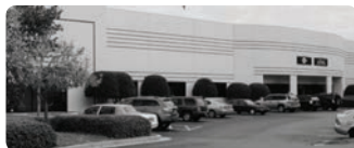
DOBLA USA MANUFACTURING LLC Office and production
