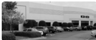
DOBLA USA MANUFACTURING LLC Office and production
